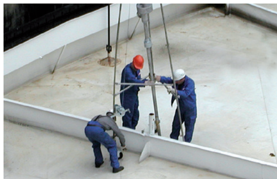
The so-called jet-washer units are installed through several liner tubes into the tank
